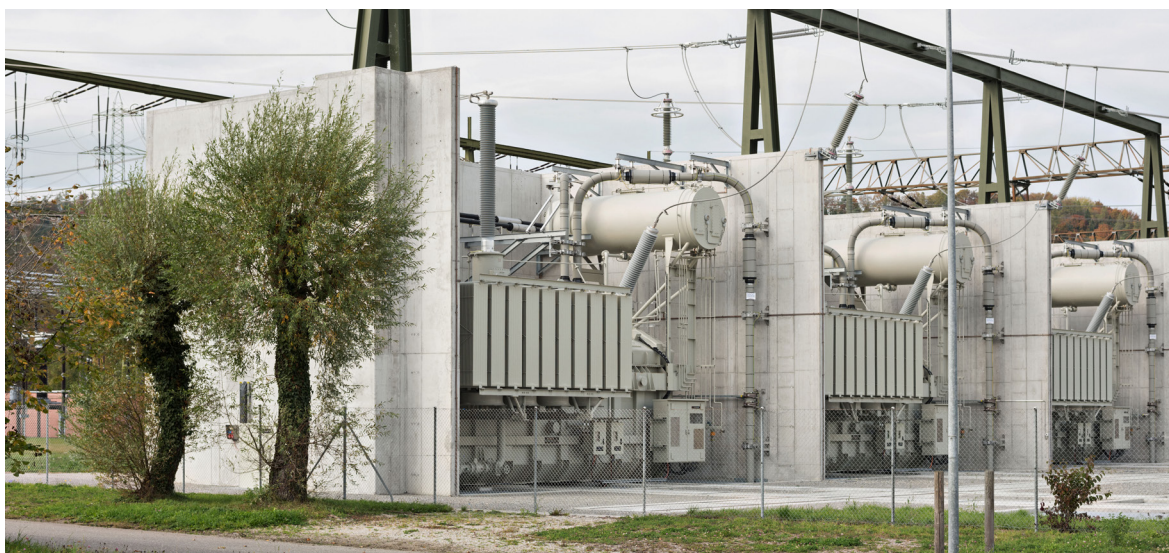
Transformers play an important role for the increasing electricity imports into Switzerland. They couple the European transmission network (380 kV) into the Swiss transmission network (220 kV). The image shows a phase-shifting transformer at Beznau substation.
