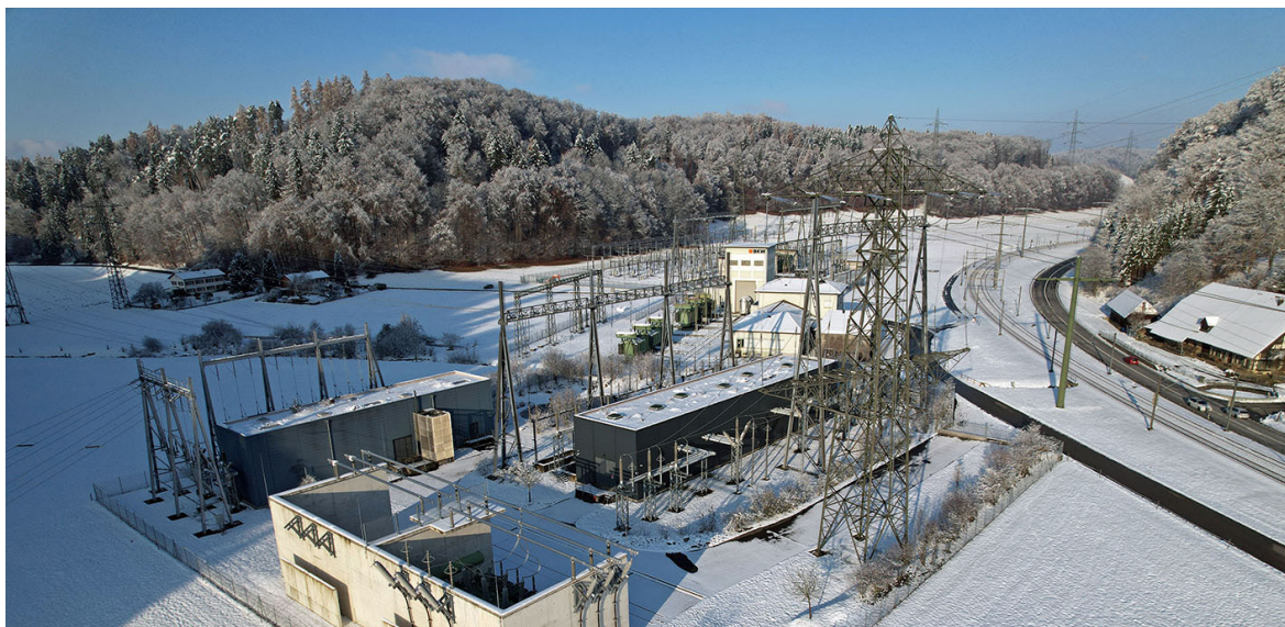
The Bickigen substation in Wynigen is one of the largest nodes in the Swiss electricity grid. Transformers here feed electrical power into the regional and supraregional distribution networks.
